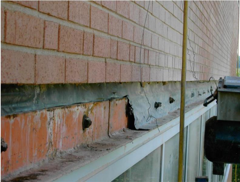
The wall opened to reveal the deteriorated flashing.
