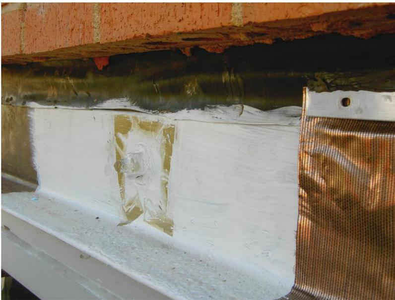
The cleaned and painted steel angle with new flashing being installed.
