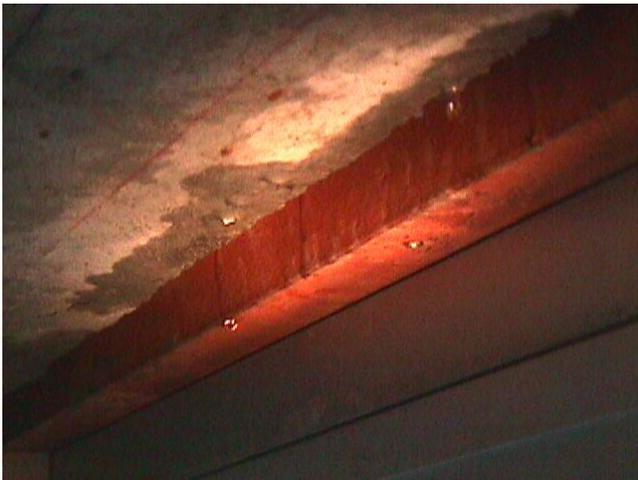
Water dripping from the wall cavity.
