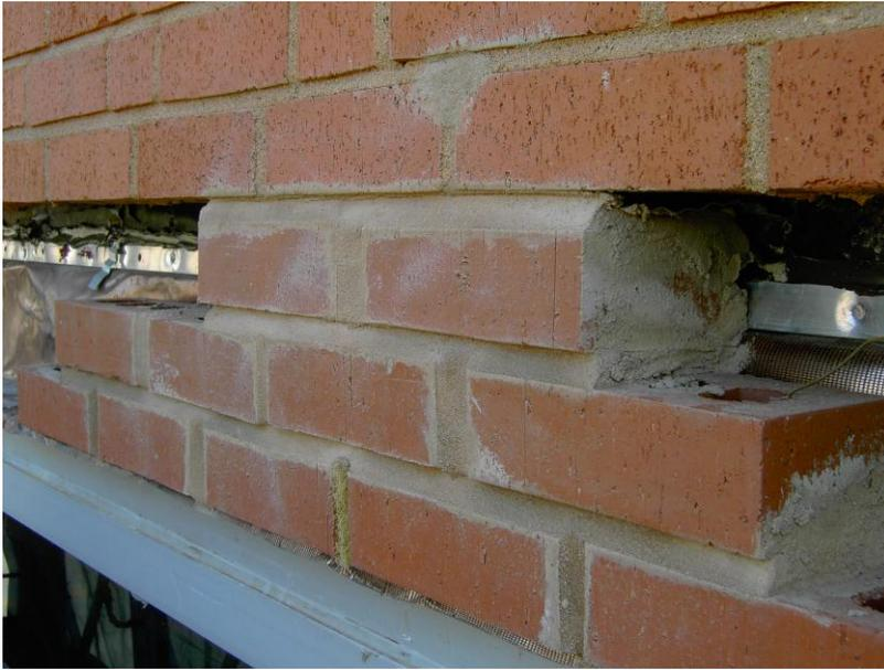
The new brick with weep holes in place of every third mortar joint.
